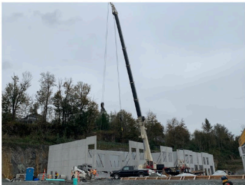
Erection of Building 3 precast walls
