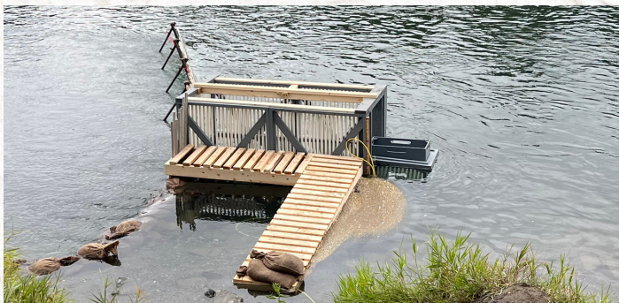
Weir Trap set up located approx. 400m downstream the Keith Wilson Bridge on the Sumas-Chilliwack River.
