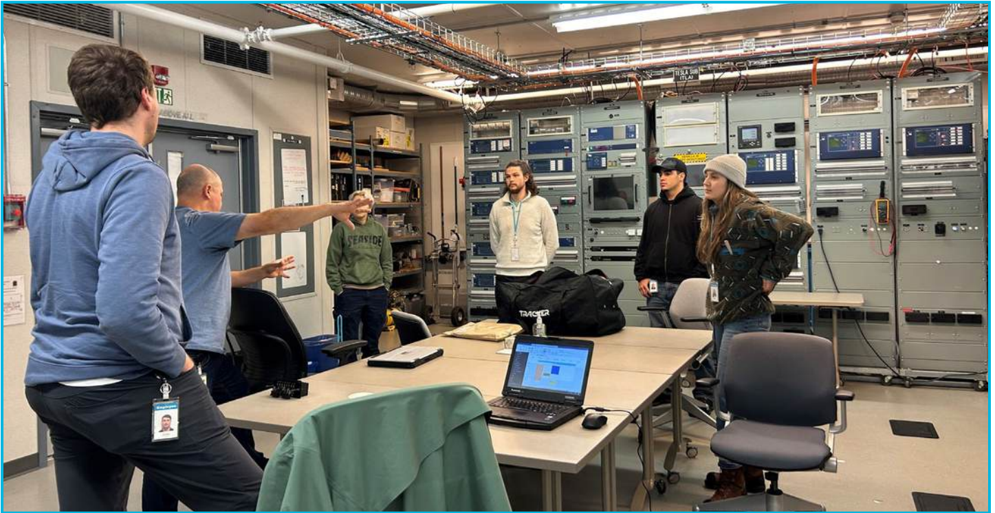
Start a career working for BC Hydro
